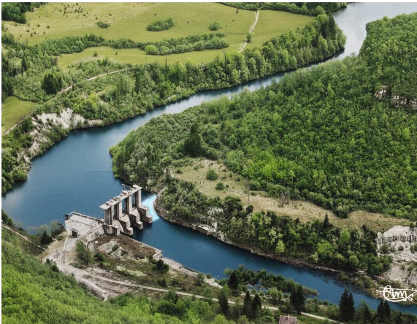
Recolorized aerial view of the Chartreuse dam and the Ain gorges before their submersion in 1968. Photo: Combier. Source: Bernard Hostache, ASPHOR.
