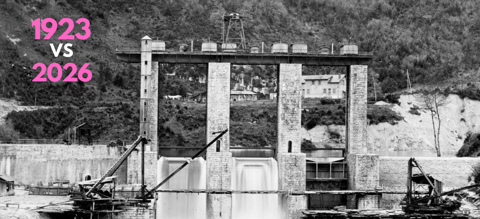
View upstream of the Chartreuse dam, with one of the gates clearly visible on the right. Source: Bernard Hostache, ASPHOR Association.
