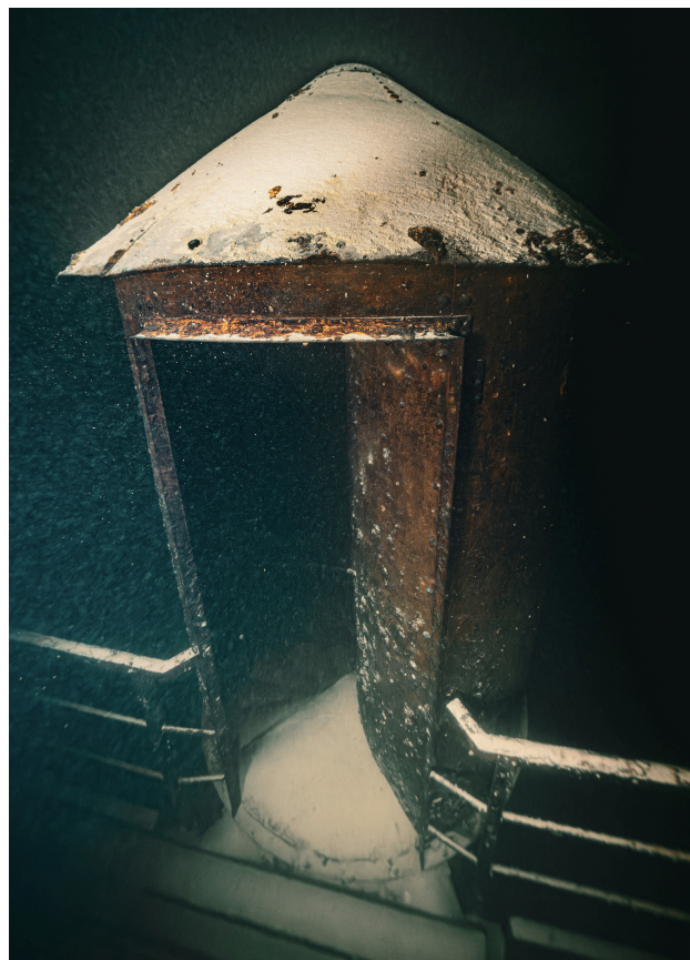
Interior of the stairwell access, located at the top of the vertical shaft. © André PiedPalmé
