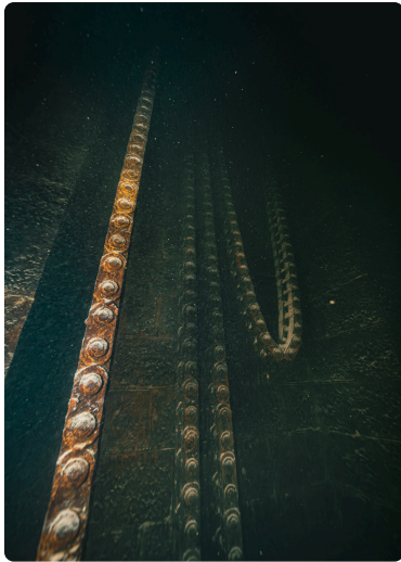
Galle chain plates of the valve lifting mechanism. © André PiedPalmé.
