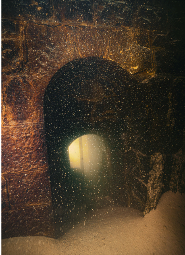
A vaulted opening at the base of a pier, set into the dressed stone masonry and passing through the structure. Against the light, one of the lifting chains can also be seen. © André PiedPalmé.
