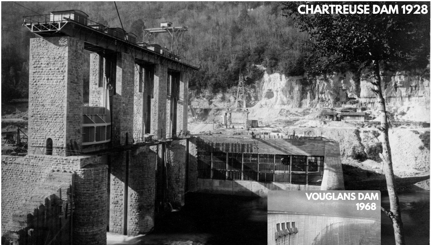
View downstream of the Chartreuse dam and its water intake (grates). Bernard Hostache, ASPHOR Association.
